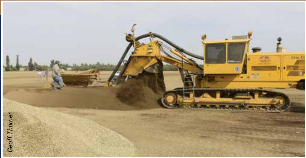
► Fresno State almond orchard groundwater recharge pipe installation, October 2020.
